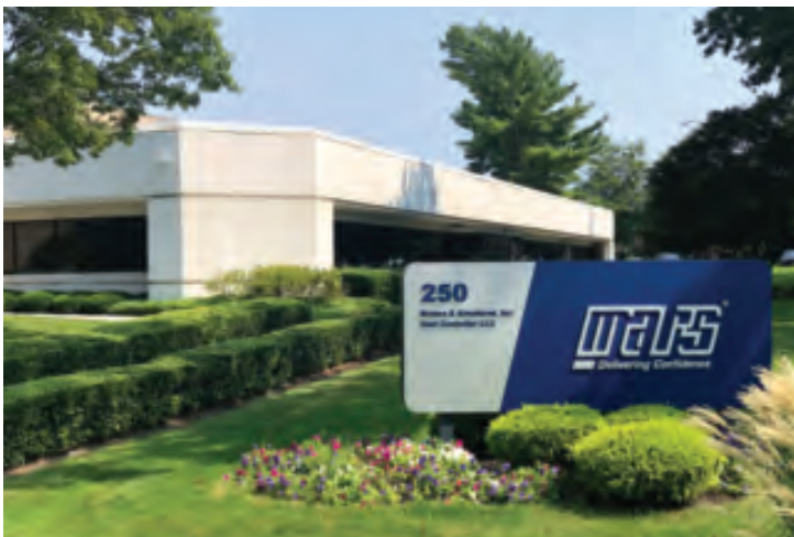
Corporate Headquarters 250 Rabro Drive East, Hauppauge, NY 11788
